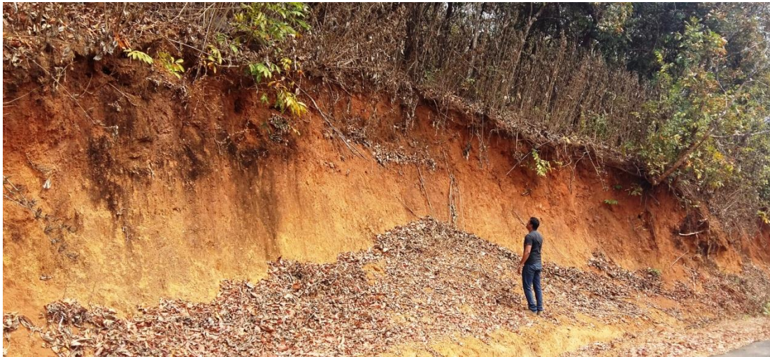
Photo: 5 Extensive road cut – Yellapur-Kaigha road
